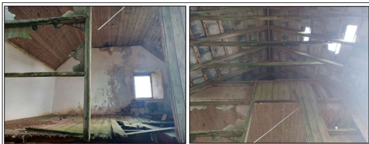
Plate 17. View of part of upper floor and roof-space of derelict cottage showing degree of deterioration
