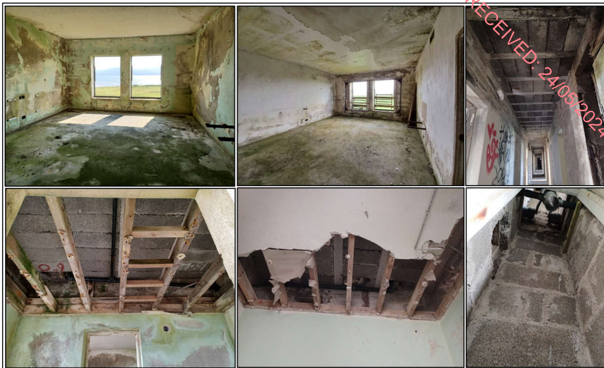
Plate 14. View of some of the more derelict parts of the bedroom block (various locations) showing examples of former bedrooms, partially/fully collapsed suspended ceilings in former bathrooms, corridors with exposed blockwork in ceilings and open shafts in internal walls
